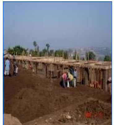
Incubator facilities under construction at KIST/CITT Remera Campus, Kigali
